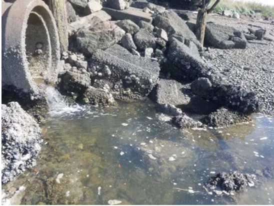
Photo of Outfall:
