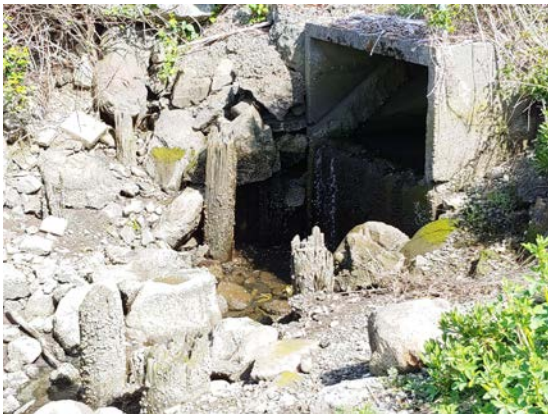
Photo of Outfall:
