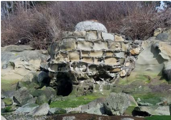
Photo of Outfall:
